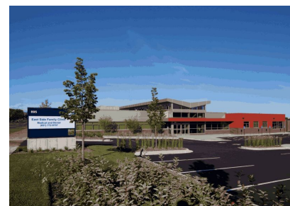
The new East Side Family Clinic in St. Paul
