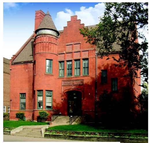
North Branch Library
